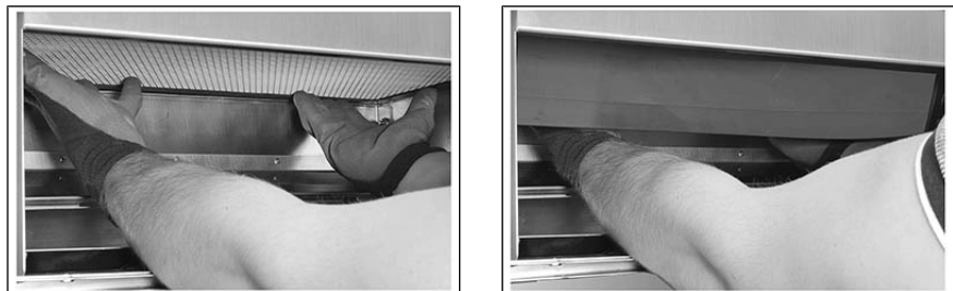
Image: Replacing the air filter
