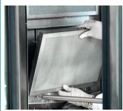
Weekly cleaning - step 1 Change the grease filters in front of the fans every three days after running the cleaning cycle. Remove a filter by lifting it up and pulling it towards you. Clean the filters in a dishwasher or let them soak in hot grease solvent for a few hours.
